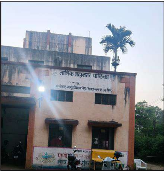
Figure 5 – Gandhinagar Water Treatment Plant
