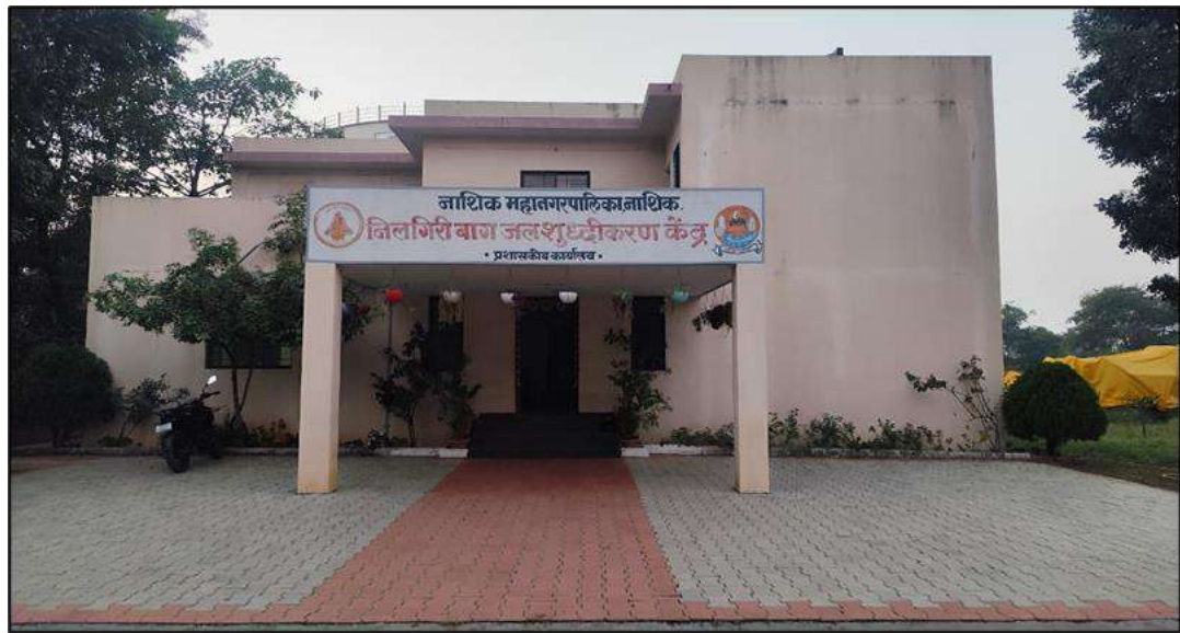
Figure 3 – Nilgiri Baug Water Treatment Plant
