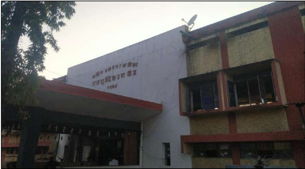
Figure 7 – Barabanglow Water Treatment Plant
