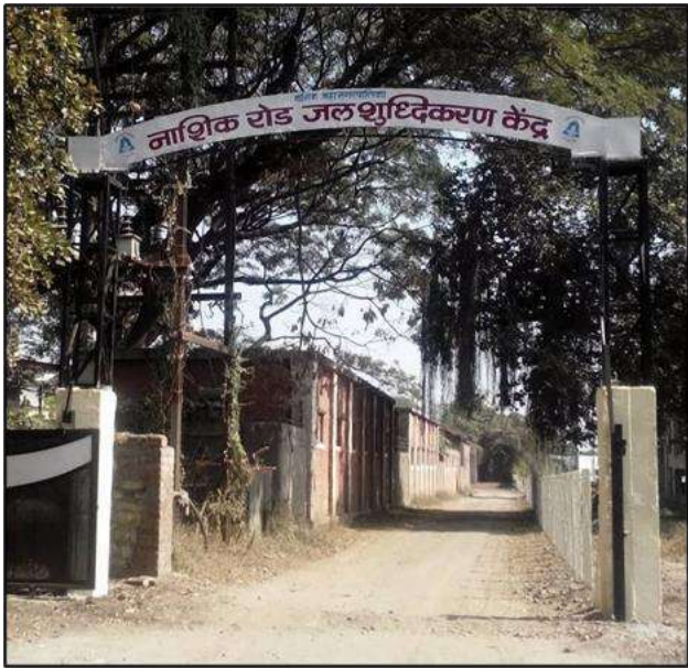
Figure 4 – Nashik Road Water Treatment Plant
