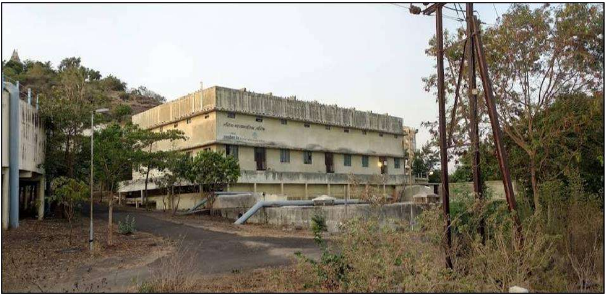
Figure 6 – Shivaji Nagar Water Treatment Plant
